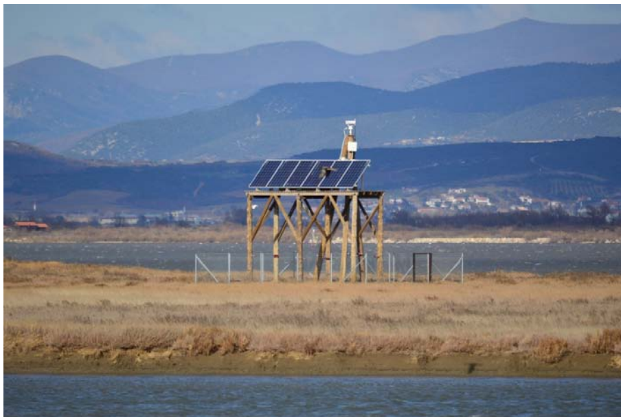
The Remote Site in Evros Delta. The system is installed on a lagoon islet, allowing access only by boat, in order to safeguard the system from vandalism. Photo: Alexandra Demertzi/HOS
