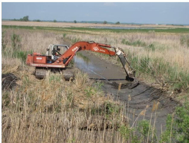
Figure 4. Channel excavation. © Dávid Bogyó/HNPD archives, May 2012
