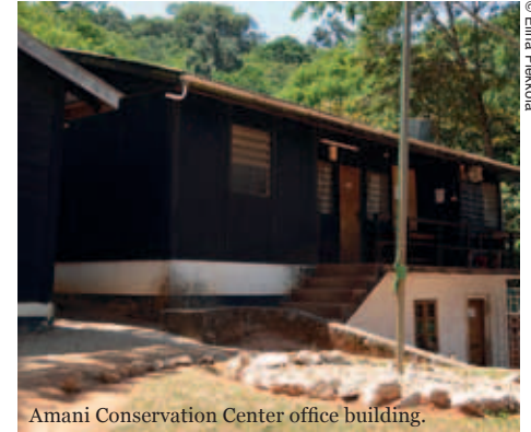
Amani Conservation Center office building.
