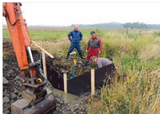
The V-dam reduces water flow and regulates the amount of chemicals.
