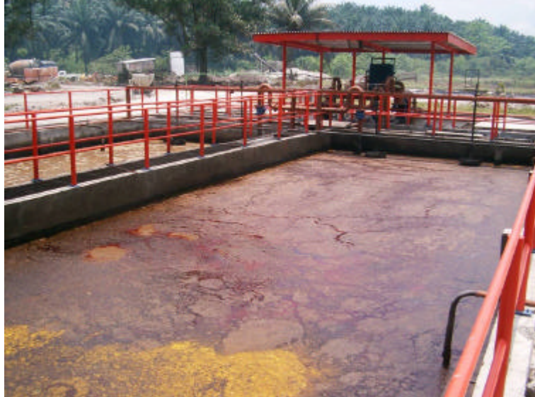
Picture 3: Effluent arising from the extraction of palm oil is temporarily stored in a cooling basin. Photograph: IFEU
