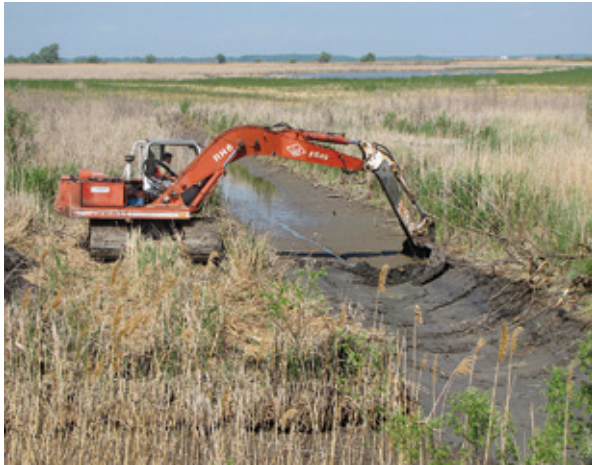
Channel excavation during May 2012. © Dávid Bogyó/HNPD archive
